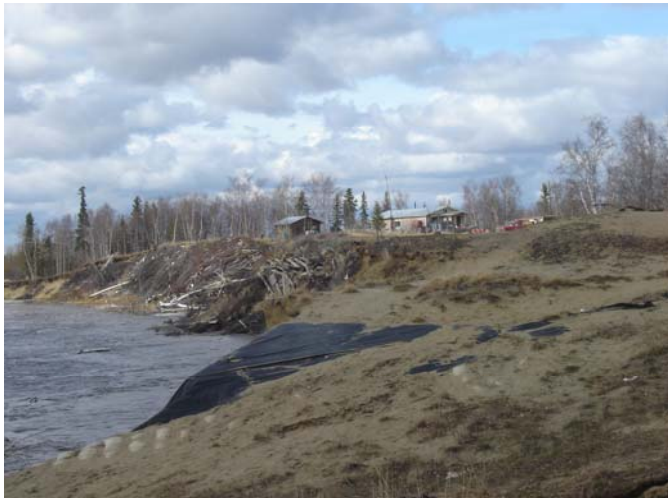
Photo 3: Koyukuk River erosion at Huslia, May 2008.
